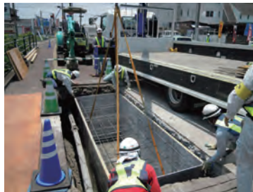
②型枠設置
